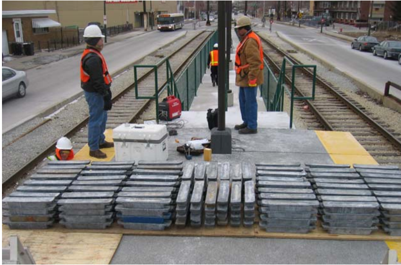
Figure 3. Full testing load of 14,160 lbs applied to the ADTP.
