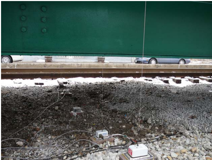
Figure 2. Cable Extension Transducers used to monitor deflections.
